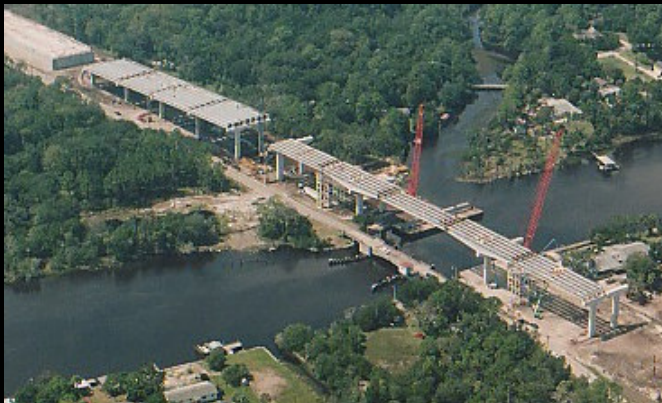
Bridge Under Construction
